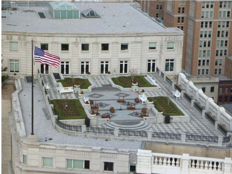
FIGURE 2.1. A recreationally-focused intensive green roof on the Evening Star Building in NW Washington, DC. Photograph by author.
