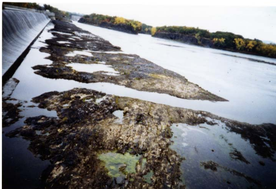
Figure 67 Outcrop below the Waterford dam [266], looking north. Peebles Island in the background (right) can be accessed, but the islands to the left not so easily.
